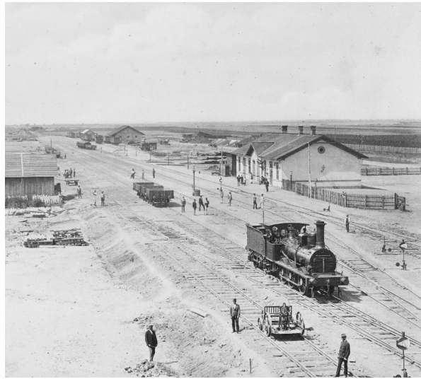
The new steam line at Trnava railway station
